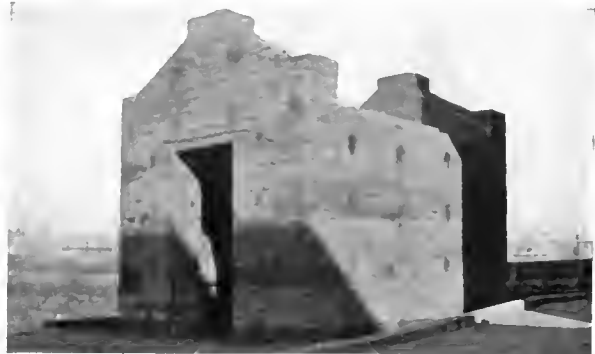
Shows completed walls ready for roof and finishing coat of plaster EARTH HOUSE, ST. LOUIS, MO. THOMAS CRANE YOUNG, ARCHITECT
